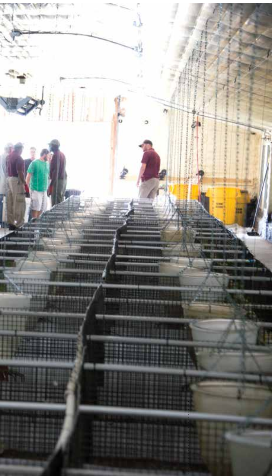
The newly renovated poultry research facility allows research and teaching programs to mirror current industry practices. (Photo by Dominique Belcher)
